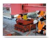
Climbing jacks are used to raise and lower heavy loads. Range from 200 to 600 ton. This kind of raising and lowering operations is carried out in steps of 10 cm
