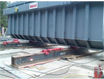
Once arrived at destination Fagioli lifted the trafo with the screw jacks in order to allow the trailer to be removed. The item was skidded with the rollers in order to align it to the tracks specially made on the foundations. Once in position, the trafo was hoisted with the hydraulic jacks allowing the Fagioli operators to place the wheels under the transformer (after the skidding beams removal). Eventually, the transformer was pushed onto tracks to its final position with winches
